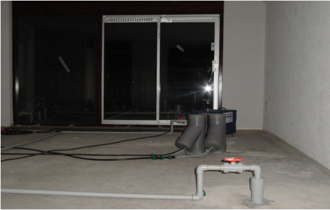
Six-Phase Heating Beneath Residential Home.
