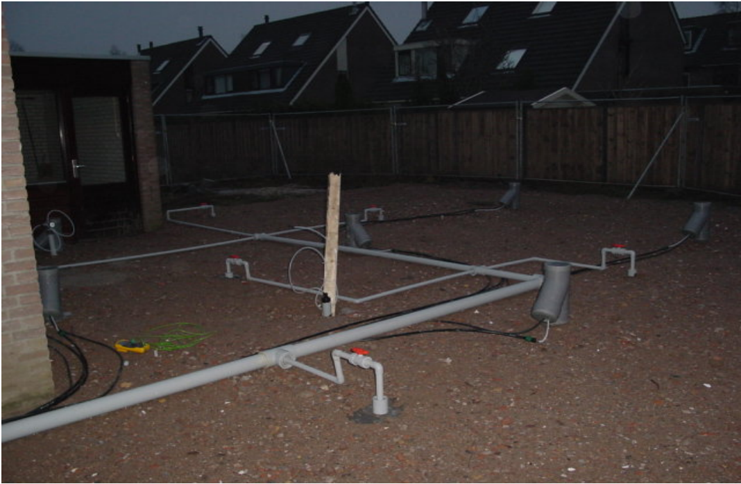
Six-Phase Heating in Residential Neighborhood. Experience only by CES
