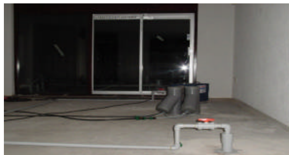
SPH Electrodes and vents beneath residence
